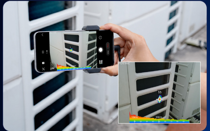
HVAC Air Leak Inspection
