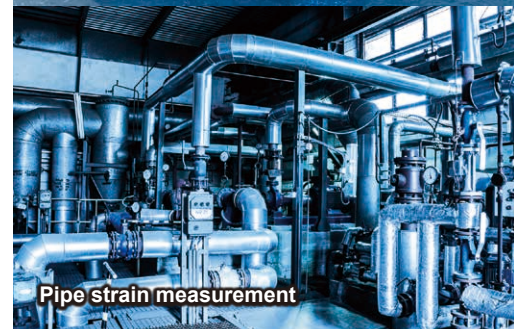
Brake and pipe strain measurement
