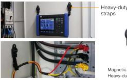
Magnetic straps can also be used to help keep voltage cords from coming loose.
